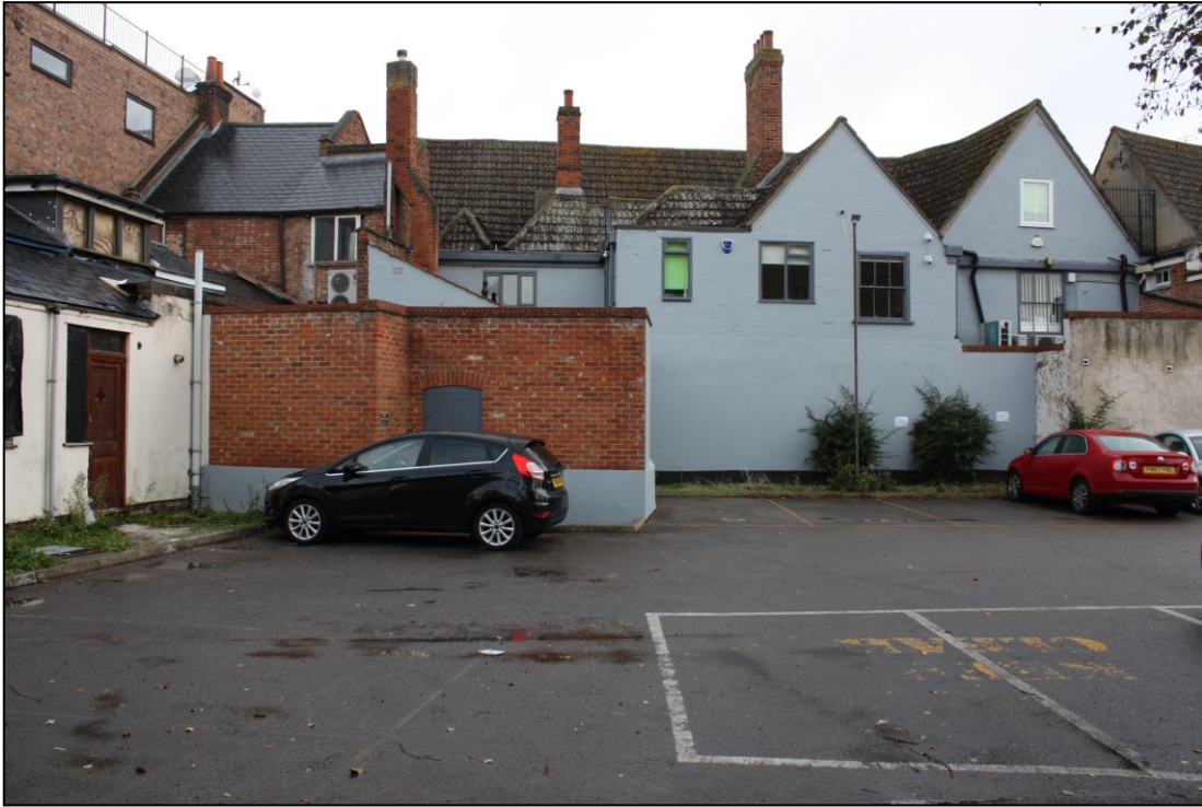
Rear of building plus parking
